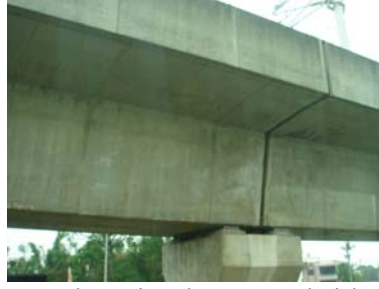
Figure 1 Overhanging beams at bridge supports
